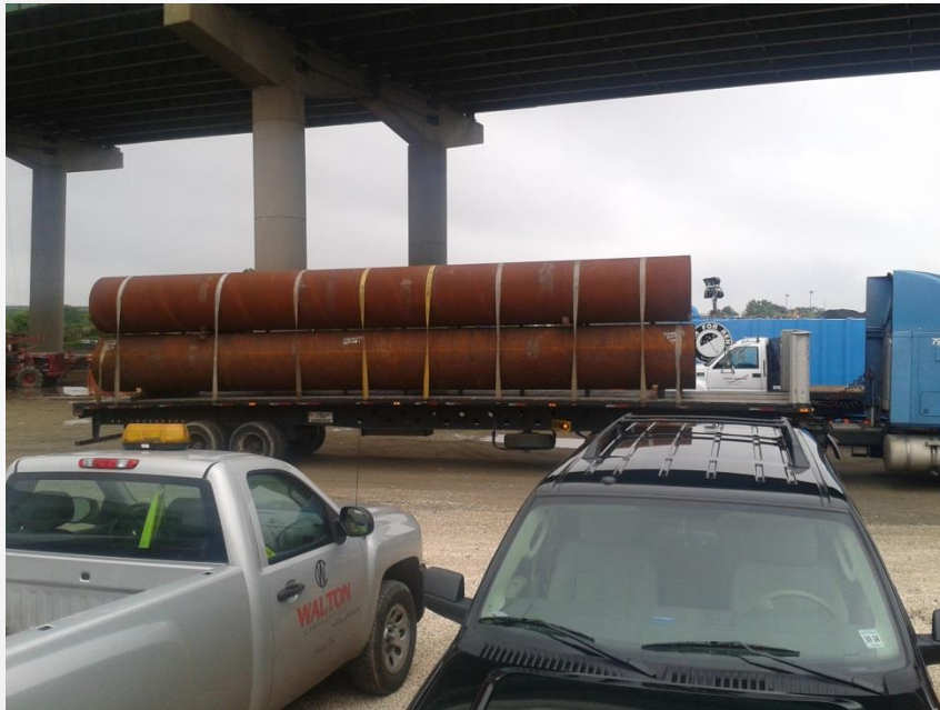
First Delivery of Casing 6/12/2014
