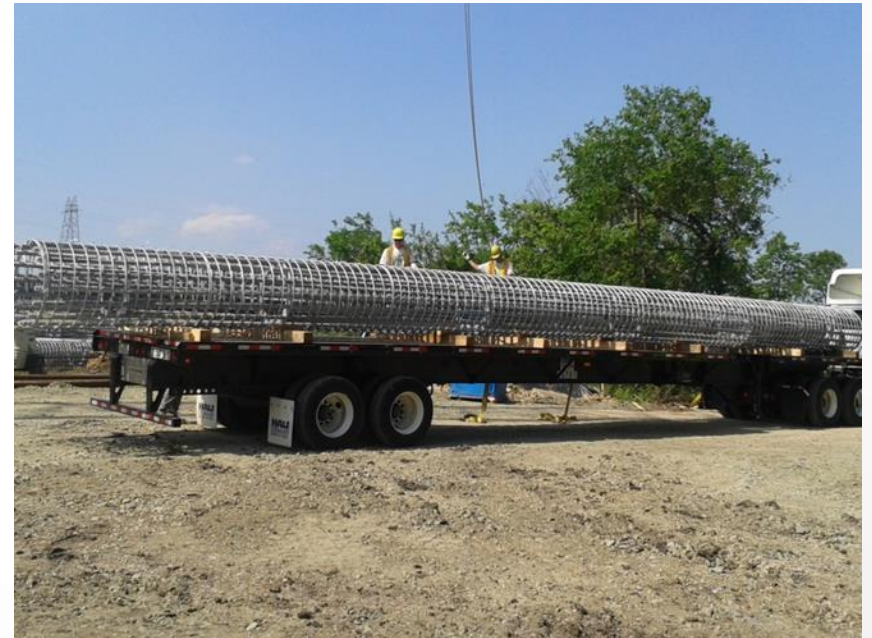
Rebar Cage from Tappan Zee project 6/16/2014
