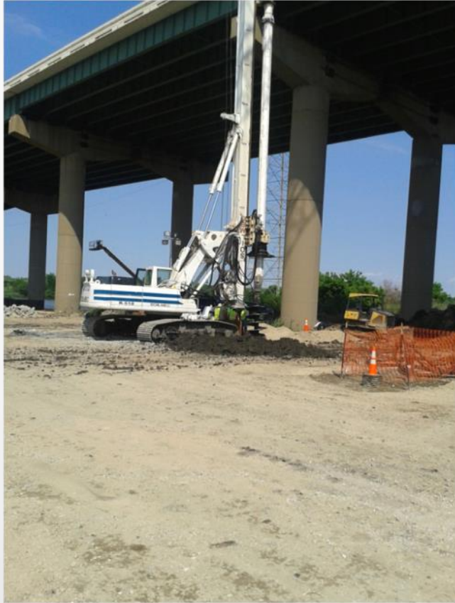
First Drill Rig on Site 6/13/2014
