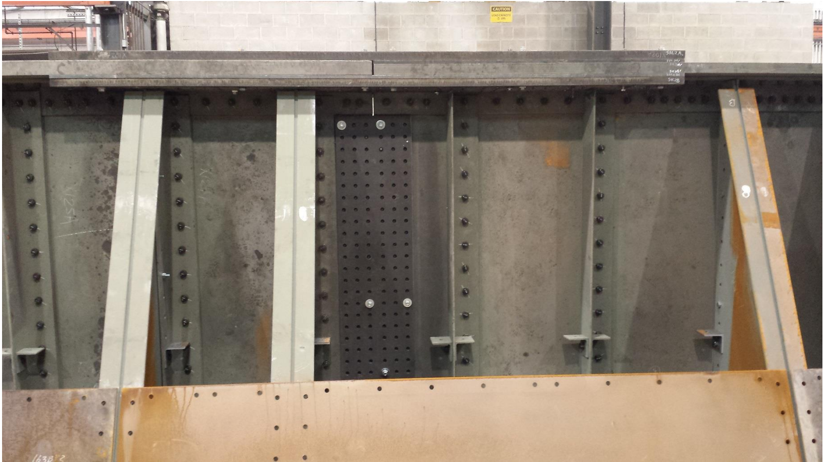
WB-207 Span 1 Field Splice
