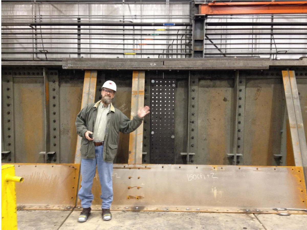
WB-207 Span 1 Field Splice
