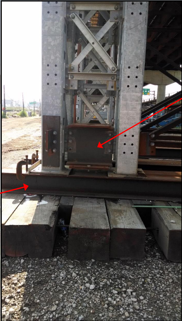
Jacking and Roller Beam
