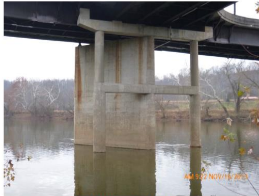
Picture 2 - Pier 3 & Pier 3A
