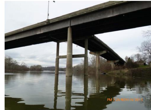
Picture 3 - Pier 3, Pier 3A and Pier 5
