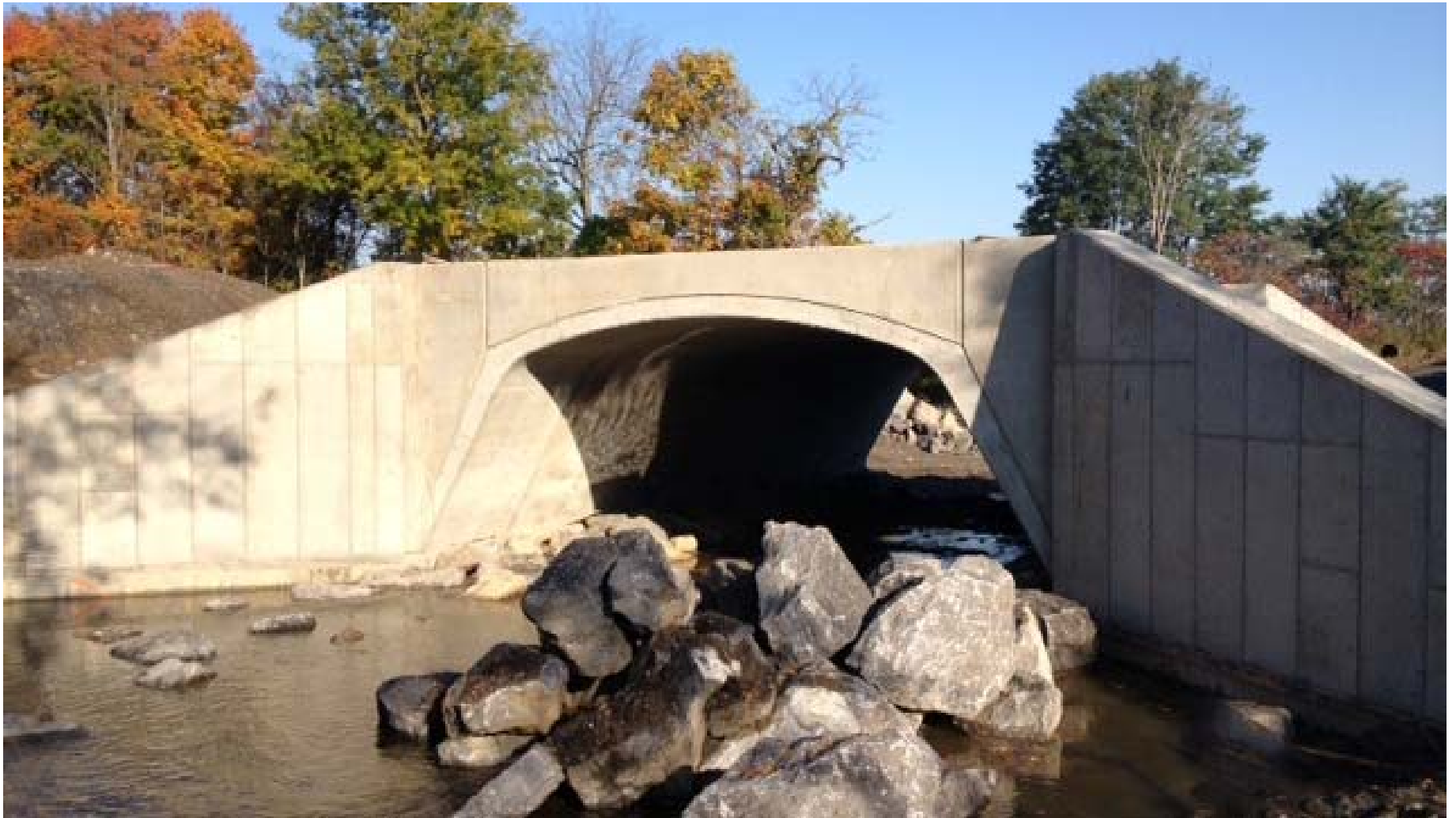
Duanesburg-Churches Road Bridge Replacement Duanesburg, New York
