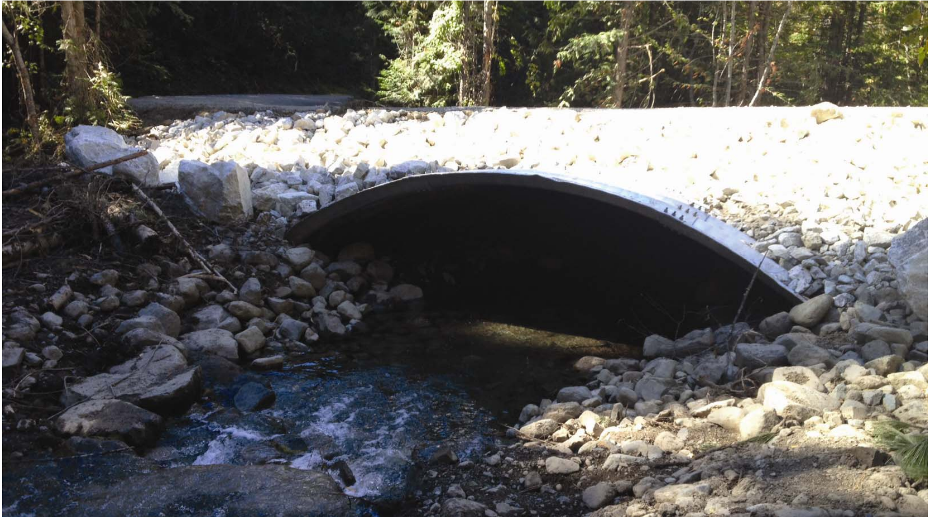
Pierre Creek Culvert Replacement Boys, Washington
