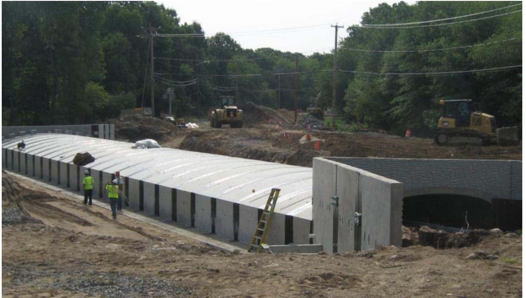
Frenchtown Brook Bridge Replacement East Greenwich, Rhode Island
