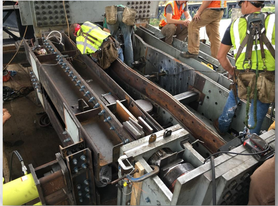
Later Jacking Stage
