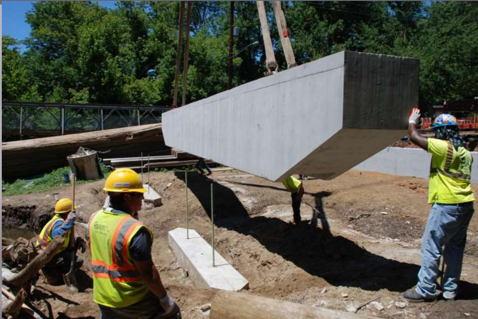
Erecting Pier Sections
