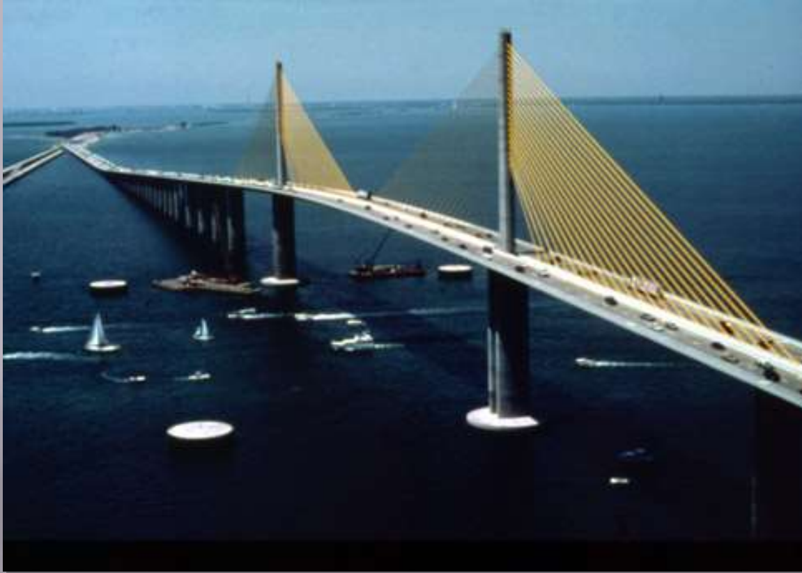
Sunshine Skyway Bridge Florida
