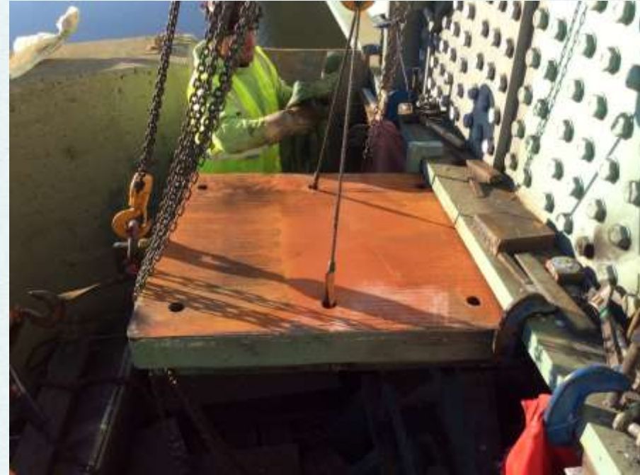
Existing Bearing Removal
