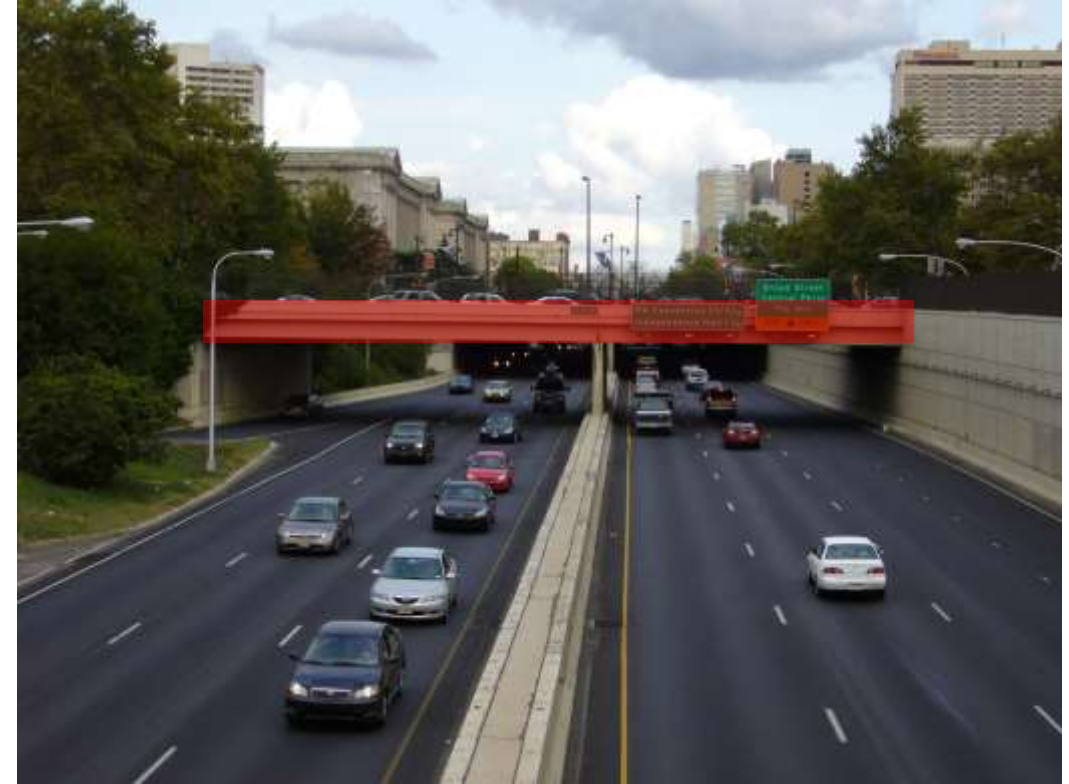
21 st Street Bridge
