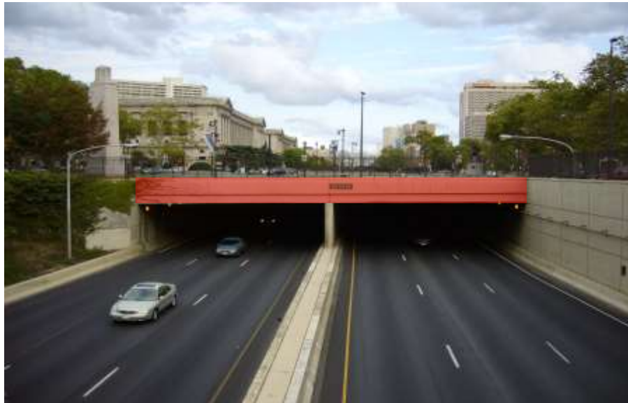
BFP/20 th Street Bridge
