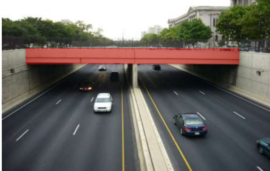
Family Court Bridge
