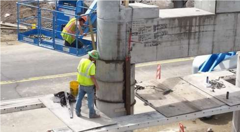
Using ready made colum steel forms
