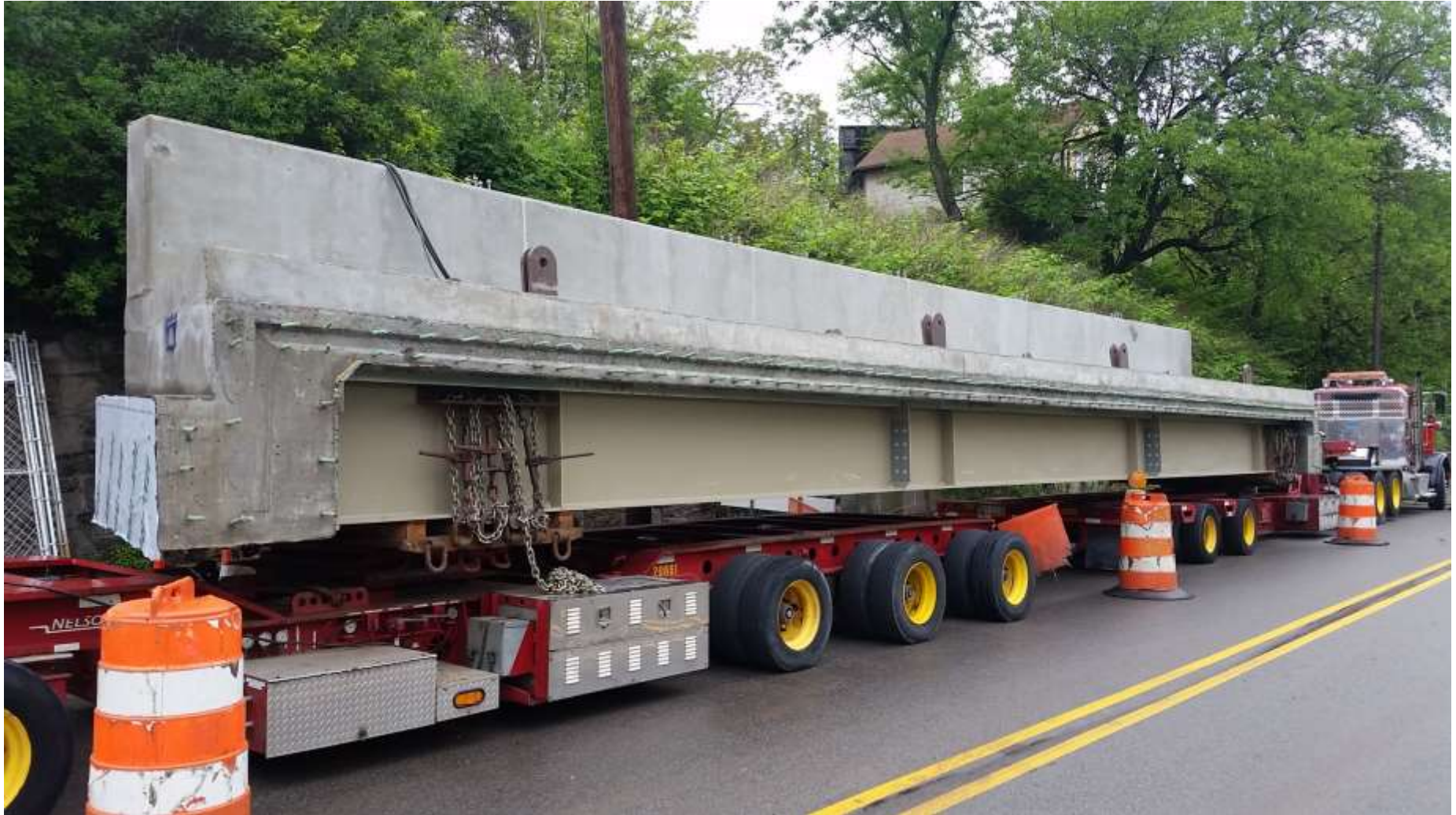
Deck Module Waiting To be Installed
