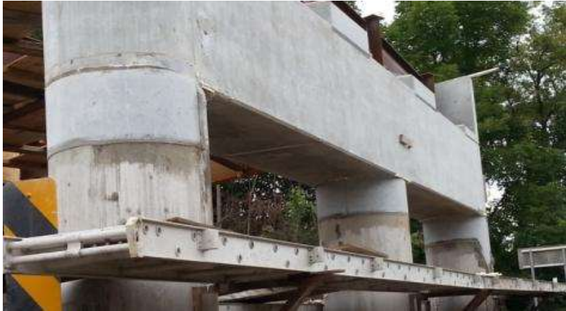
Completed repair before painting
