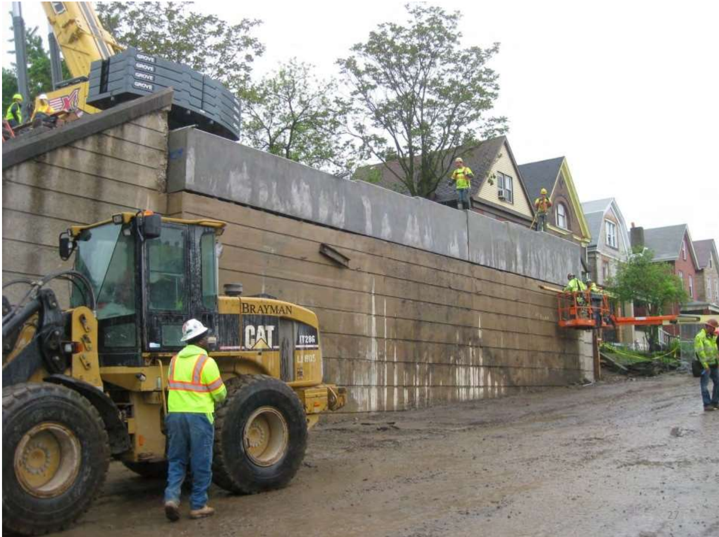
East End Precast Abutment Cap In Place
