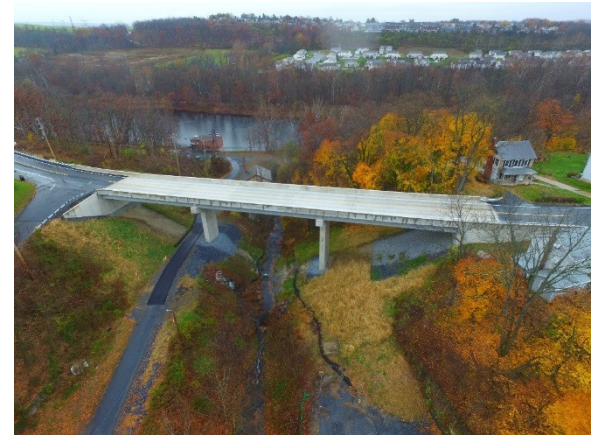
SR 1027, Spring Creek Bridge Replacement, Lehigh County, PA Michael Baker International, Inc.
