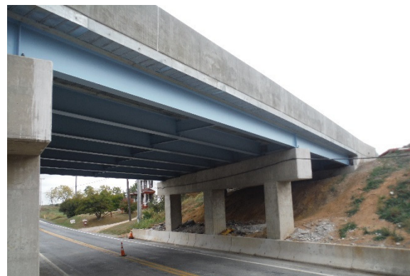
I-81 Bridges over Leitersburg Road, Franklin County, PA Borton-Lawson
