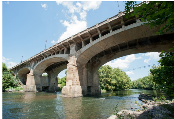
Schuylkill Avenue Rehabilitation, City of Reading, PA Michael Baker International, Inc.
