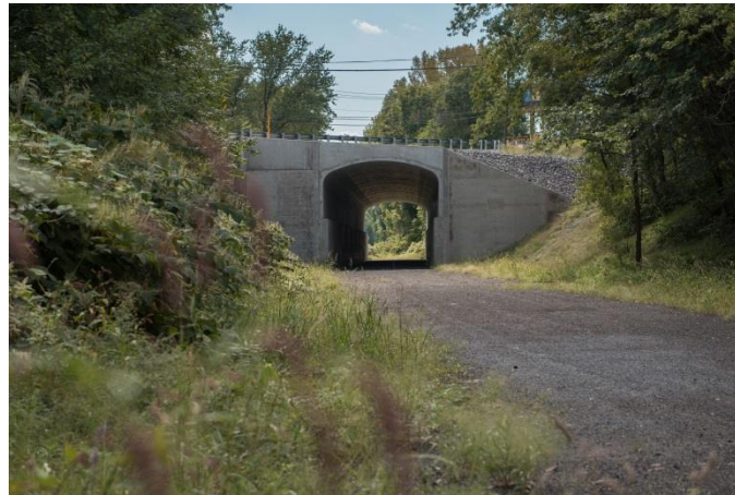
State Route 11 Bridge, Luzerne County, PA RETTEW
