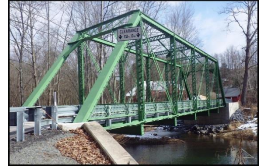
Little Muncy Creek Pratt Truss, Lycoming, PA Dewberry Engineers, Inc.
