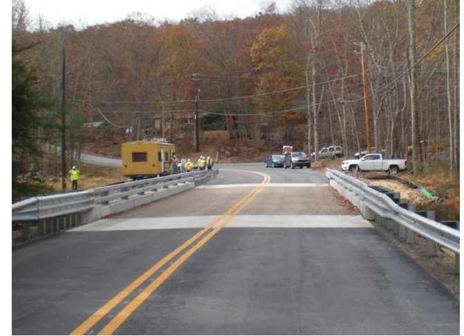
Snow Hill Road Bridge, Monroe County, PA Century Engineering, Inc.
