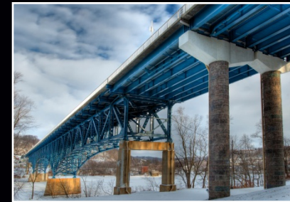
Freeport Bridge Rehabilitation over the Allegheny River Modjeski and Masters, Inc.
