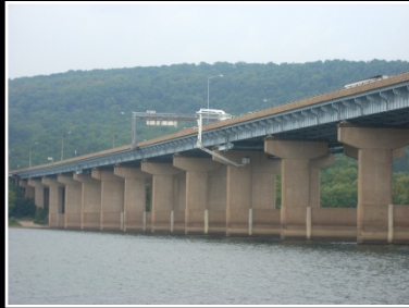
George N. Wade Bridge (SR 0081, Section 042) over Susquehanna River & Norfolk Southern RR tracks Gannett Fleming, Inc.
