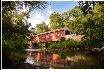
Siegrist Mill Covered Bridge Restoration RETTEW Associates, Inc.
