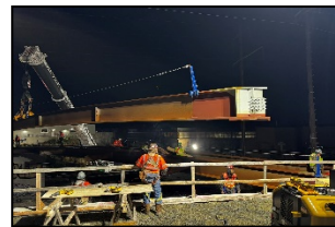
Medium Span Category Montgomery Avenue Bridge, Modjeski and Masters, Inc.
